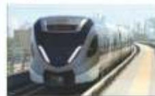
DOHA METRO ROLLING STOCK & TRUCK WORK - PHASE I SYSTEM
